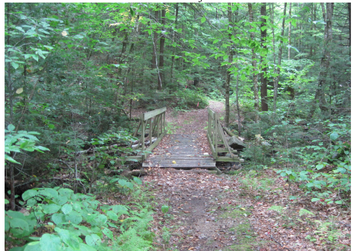
One of several bridges on the Kilburn Trail
